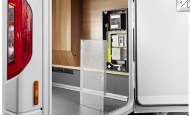
Electrical centre easily accessible in scooter garage
